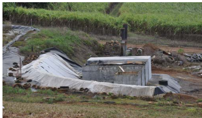
Hazardous waste cell at Mare Chicose landfill
