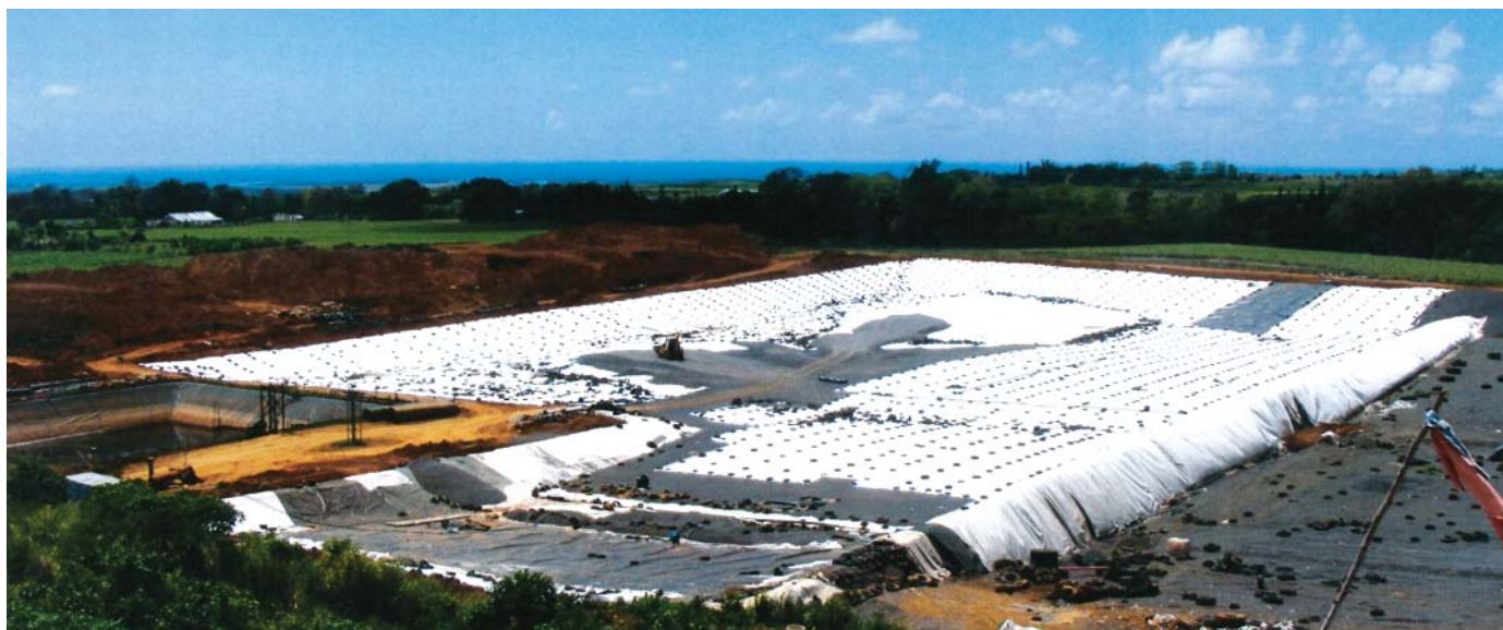
New waste cell at Mare Chicose Sanitary Landfill (Courtesy: Ministry of Local Government & OI)
